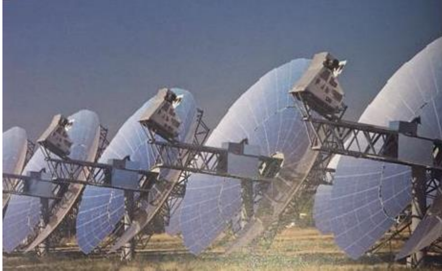
Figure 6. An array of 60 parabolic dishes each with a 25 kW Stirling engine constructed at Maricopa in Arizona in 2010
