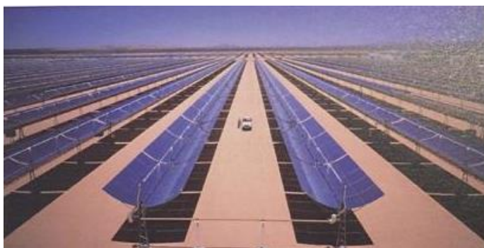
Figure 4. SEGS solar collector field at Kramer Junction in southern California
